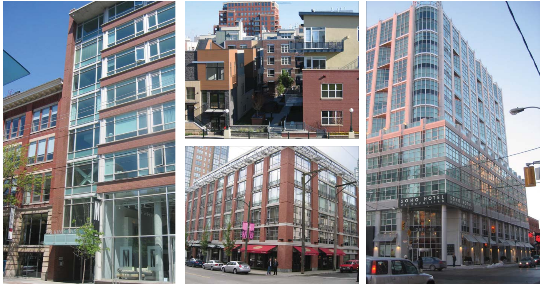
The examples above demonstrate some key characteristics of redeveloped urban infill blocks: (clockwise from the top) an urban infill site responds to a variety of surrounding conditions with buildings that vary in scale; a 16-story hotel / condominium locates active uses at grade; a modern mixed-use infill project with retail at-grade; an infill project with a modern aesthetic while incorporating materials similar to an adjacent historic brick structure.
